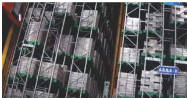
Automatic Storage and Retrieval System (ASRS)
