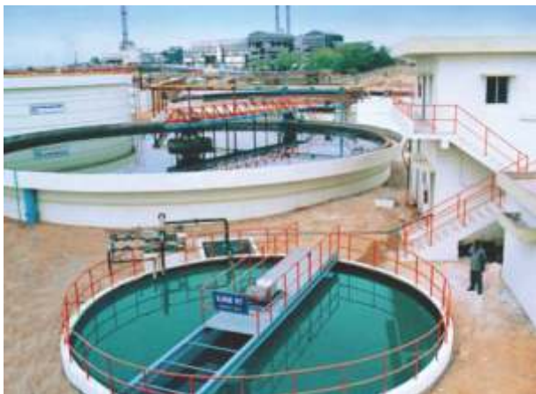
State of the art Bio-methanation plant
