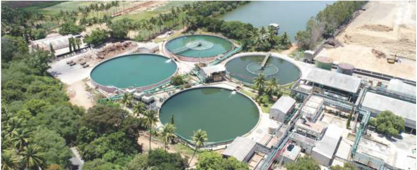
Waste water treatment plant
