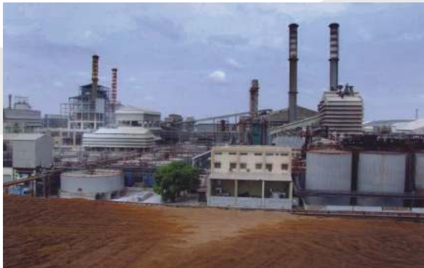
View of TNPL mill from bagasse yard
