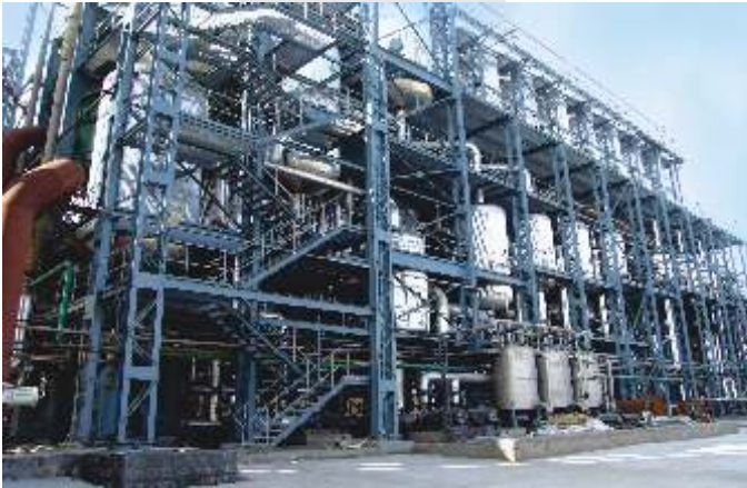
350 TPH Black Liquor Evaporation Plant
