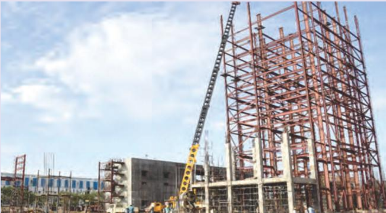
Mill Expansion Plan of Unit II - Erection of Chemical Recovery Boiler in progress
