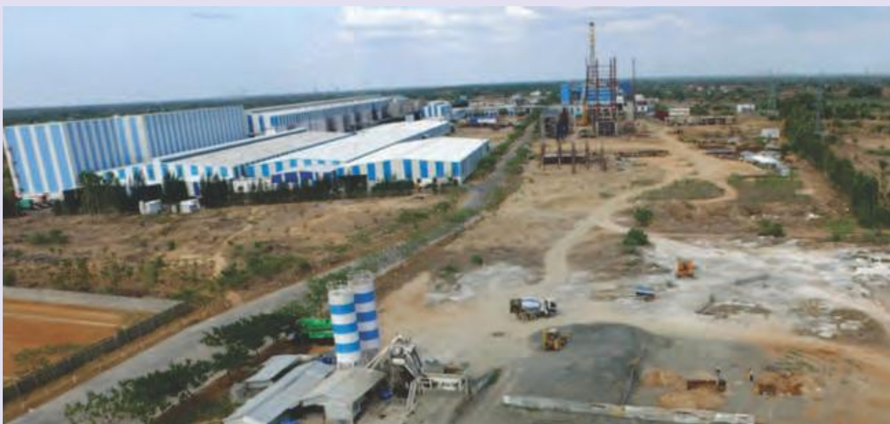
Project Site - Mill Expansion Plan in Unit II under implementation
